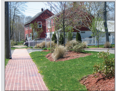
"brick" stamped sidewalk at Stage Road
