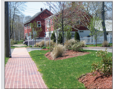
"brick" stamped sidewalk at Stage Road
