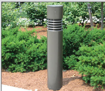
pathway lighting at the Town Hall
