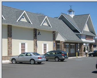
parking aisle with two outlets
