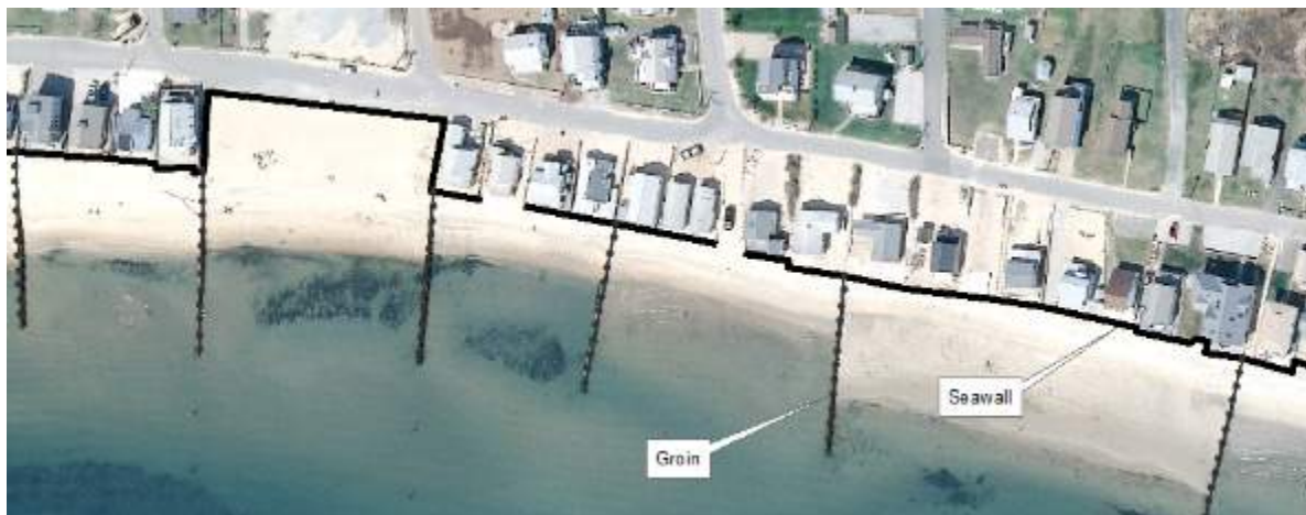
Figure 6: Groins and hardened structures along shoreline, Chalker Beach
