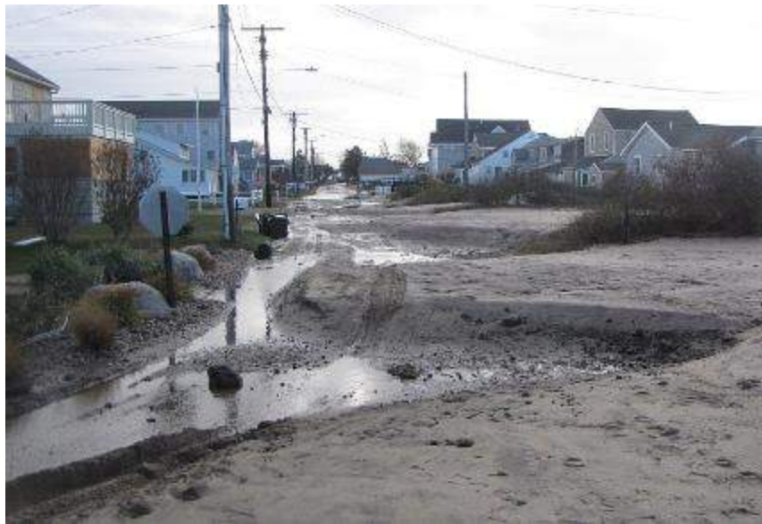
Figure 23: Not only flood waters but sand can make roads impassable; Beach Road West following Storm Sandy
