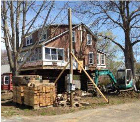
Figure 21: House being elevated, Sea Lane
