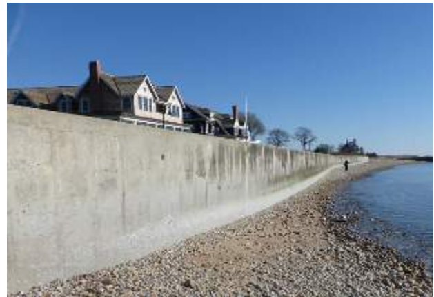
Figure 5: Seawall located in Fenwick
