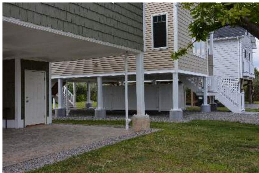
Figure 22: Recently elevated houses
