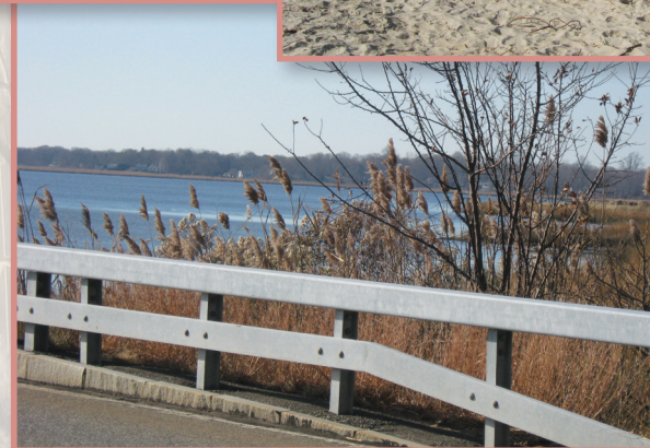
Context sensitive guiderails and granite curbing do not detract from the view and keep vehicular traffic safe.
