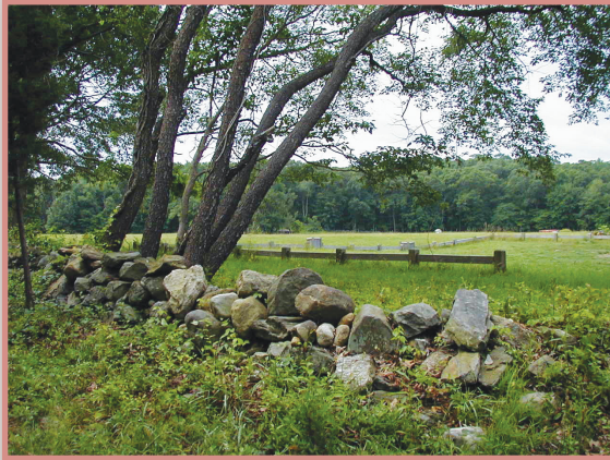
View of open field is maintained by clearing underbrush in front of stone fence.
