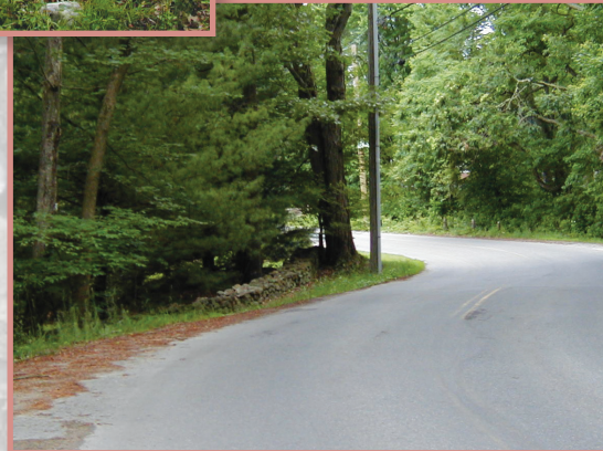
Narrow pavement lies within the Ingham Hill Road right-of-way.
