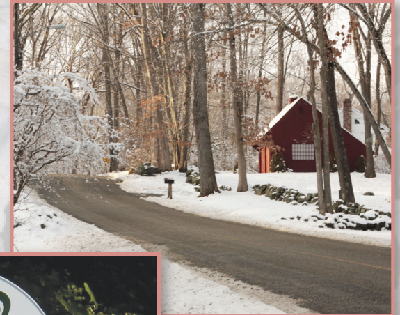
Narrow pavement lies within Schoolhouse Road right-of-way.
