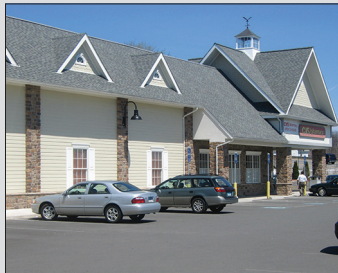
parking aisle with two outlets
