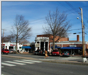
Main Street Crosswalk
