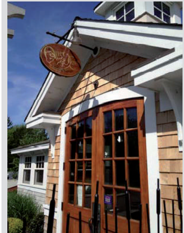
Front door detail on Essex Road
