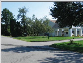
bank kiosk accessed from Orchard Street
