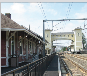
Saybrook Junction and Estuary Transit District
