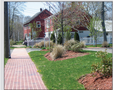
"brick" stamped sidewalk at Stage Road
