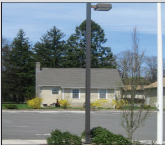
parking lighting on Boston Post Road East
