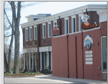
second-story windows sized for future residences
