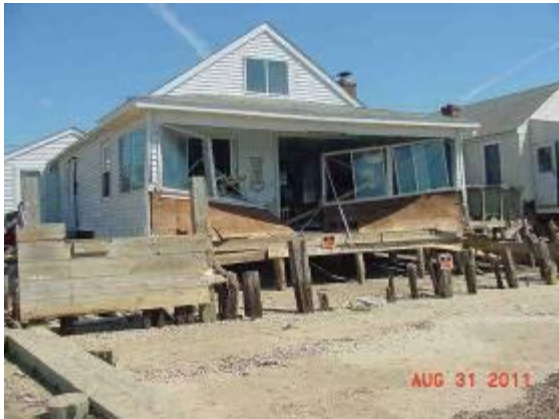
Figure 8: 2011 Tropical Storm Irene damage - Damaged house on Beach Road.
