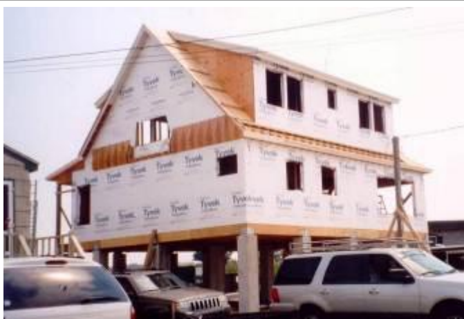
New home construction. New homes built in coastal areas of Old Saybrook must comply with current building code requirements for flood elevation and high winds and must comply with the Town's Flood Ordinance which now requires 1' of freeboard above the FEMA base flood elevation.
