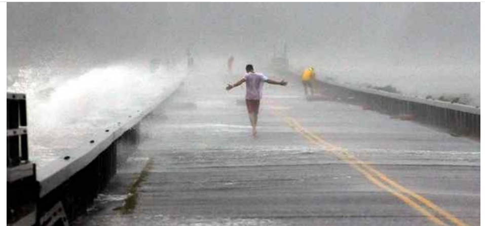
South Cove Causeway during Irene showing wave overtopping bridge deck. This photo, by Mara Lavitt, won a first-place award in the Connecticut SPJ contest. "Thrill seekers on the causeway between Old Saybrook and Fenwick Point during Tropical Storm Irene, on Aug. 28, 2011." The tide gage data indicated a peak water level during Irene of about Elevation 6.5 feet NAVD (about or slightly higher than the bridge deck elevation). In comparison, the same tide gage measured a peak water level of about Elevation 8 feet NAVD during Sandy.
