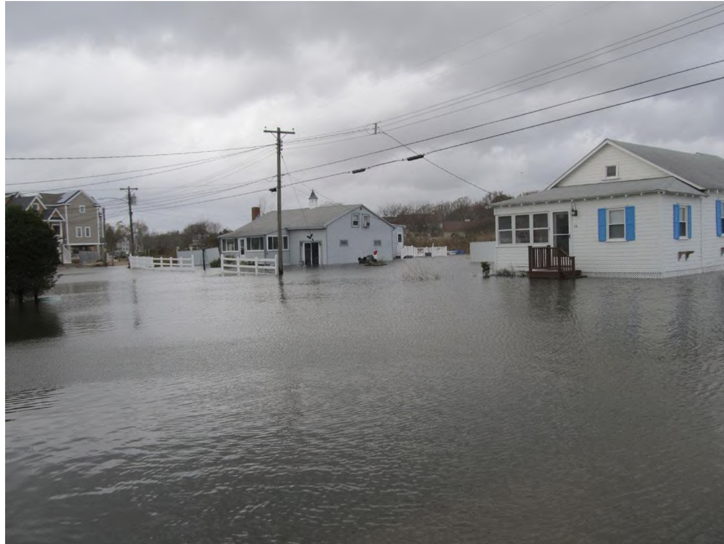
Street flooding in Chalker Beach following Sandy )(mage from https://ctmirror.org/ )
