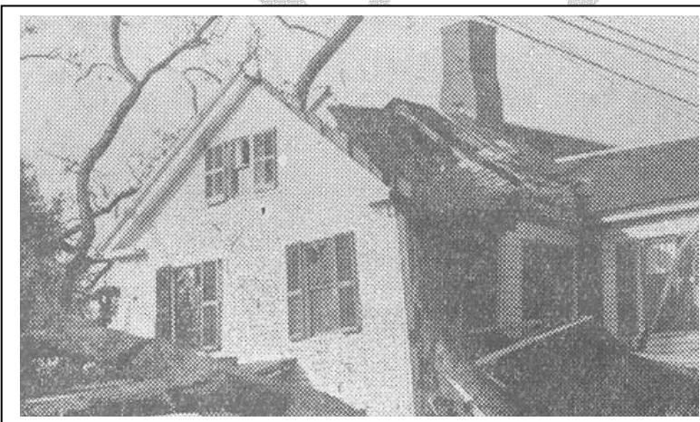
Figure 7 - Significant damage occurred inland from wind during the 1938 hurricane
