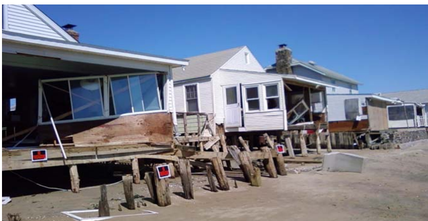
Figure 10: Coastal Storm Damage Examples of damage at Chalker Beach caused by Tropical Storm Irene, September, 2011.
