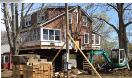
Sea Lane house being elevated above FEMA Flood Elevation
