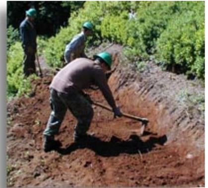
Three major factors work together to ruin a trail. First, mud and other debris slide down onto the trail. This is called **slough**. Slough blocks or narrows trails. Second, plants growing along the outside edge of the trail cause the formation of **berms**. Berms trap water on the trail leading to erosion. Lastly, trail users whether wheels, hooves or boots wear down the tread with heavy use.
