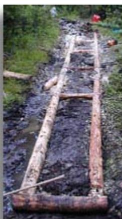
Big mud-holes or boggy areas are ideal locations for a **turnpike**. A turnpike is an elevated walkway constructed of two parallel logs or rock walls filled in with rock and **mineral soil**.
