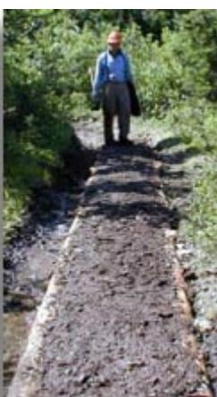
Fill the turnpike with large, flat rocks as big as you can carry, but not so large that they stick up higher than the logs. Next fill the turnpike with smaller rocks and then even smaller rocks filling in the empty spaces between larger rocks as you go. Finally fill the turnpike with fine mineral soil putting enough to form a crown higher than the logs on either side. This will keep water from pooling in the turnpike.
